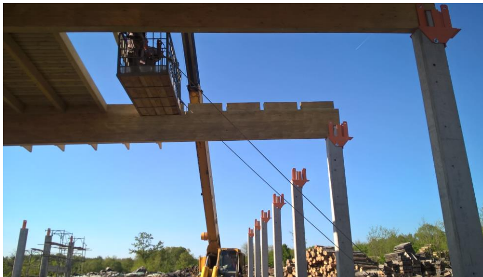
Figure 8. Erection of timber structures of industrial hall „B”
