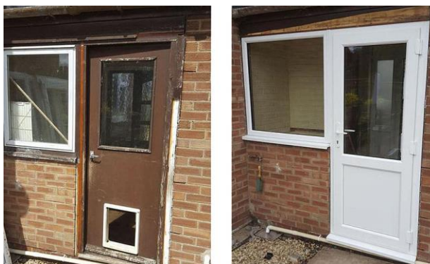
Figure 6: Replacement of old window and door frames [5]
