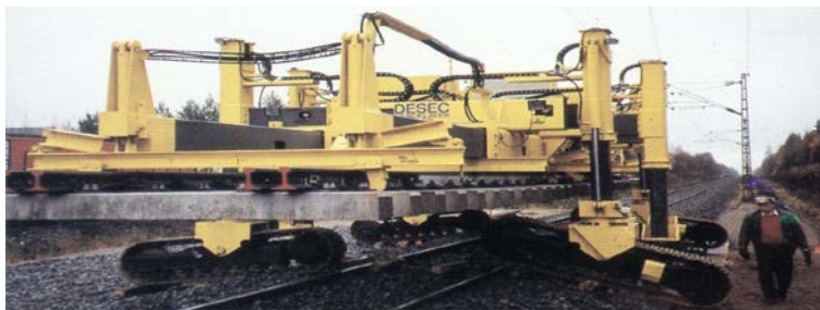
Figure 9 - DESEC crane for laying tracks and switches [5] Figure 9 - DESEC kran za polaganje koloseka i skretnica [5]
