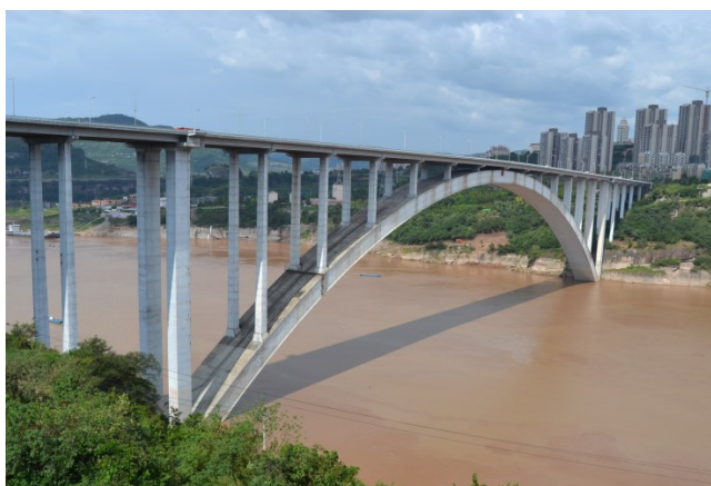
Figure 4. Wanxian bridge, Wanzhou, Chongqing, China (1997.) [25]
