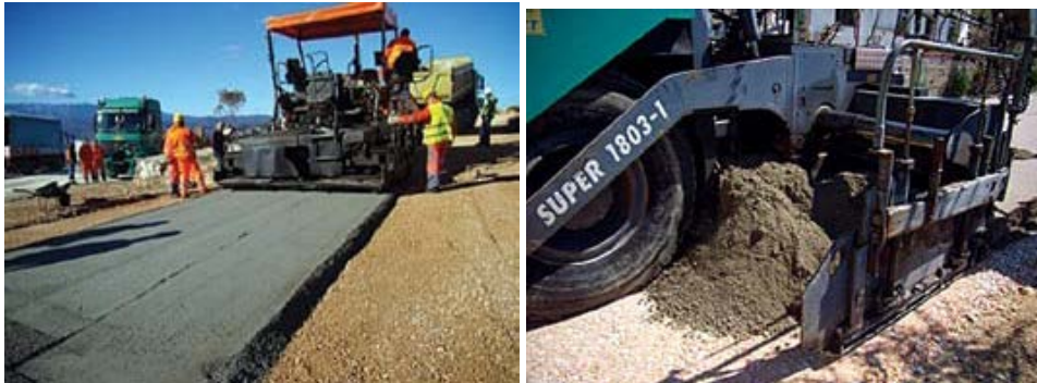
Figure 6. Installation of RCC using asphalt paver [3]
