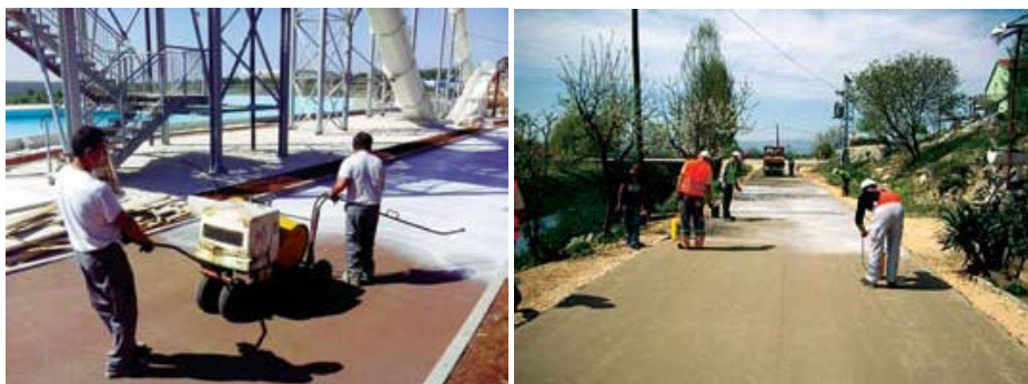
Figure 10. Care of RCC with chemicals [3]
