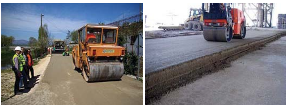
Figure 7. Compaction of RCC with roller [3]
