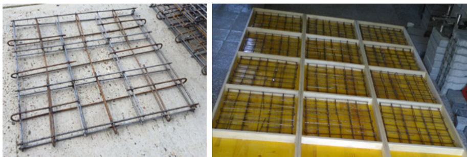
Figure 2: Reinforcement and formwork of concrete panels
