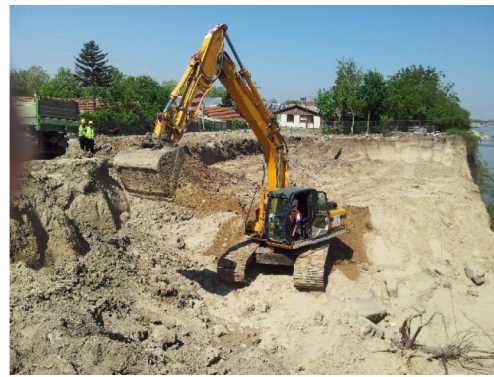
Fig. 2(b) Tracked excavator (bagger)
