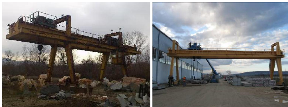
Figure 1. Original state of the crane (left) and newly constructed state (right)
