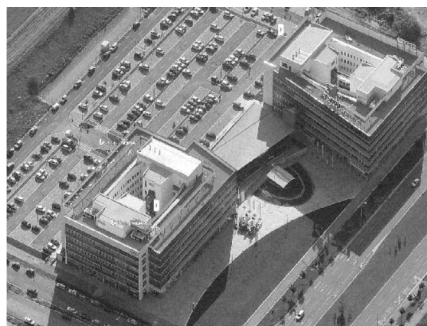
Fig. 2 - GTCS Buildings: C, A, B
