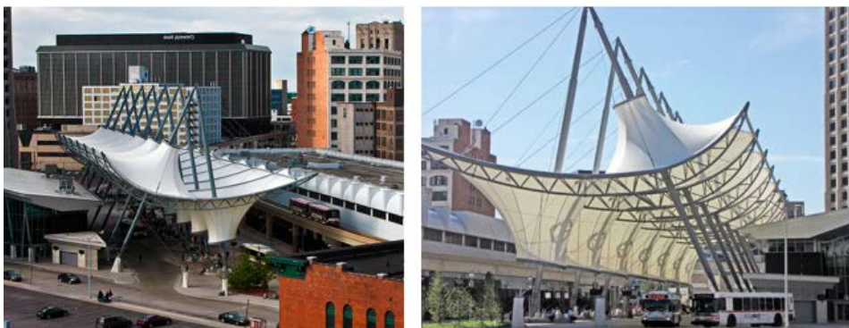
Figure 5. Rosa Park Terminal in Detroit [10, 11]
