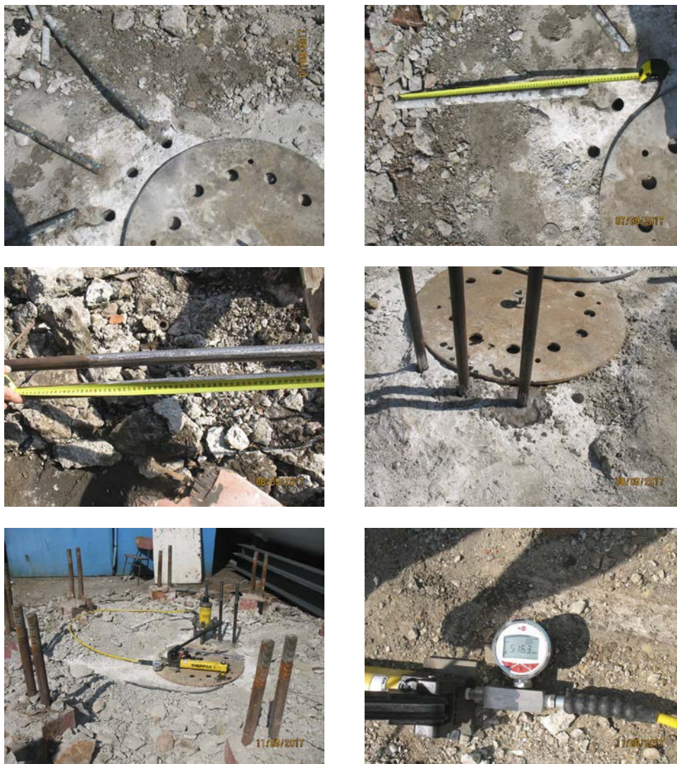
Figure 4. Testing of the anchor bolts
