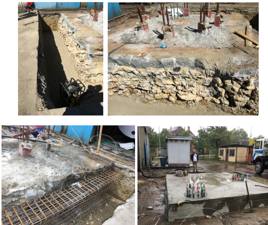
Figure 7. The restored foundation with new anchors
