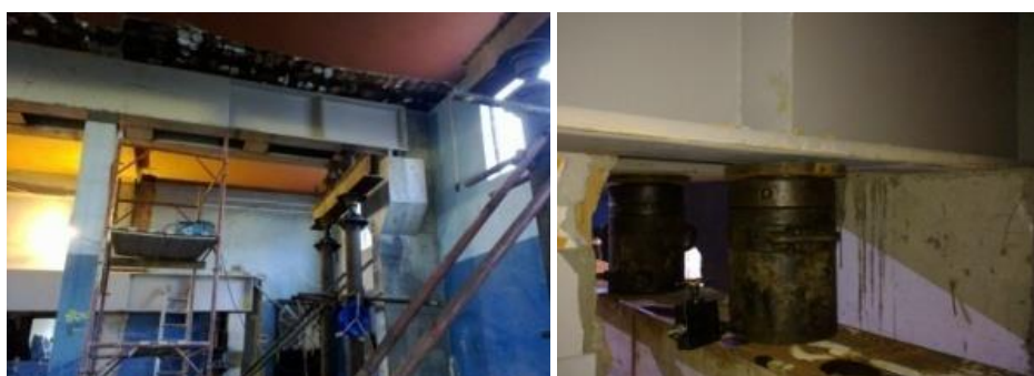
Figure 12. Lifting of steel girders by hydraulic presses
