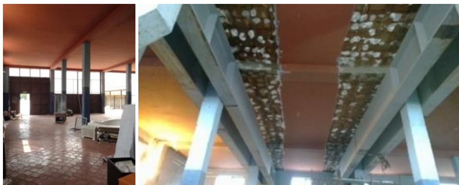
Figure 11. Existing columns for demolition and new steel girders
