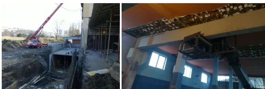
Figure 10. Excavated basement and placing of the steel I-beams
