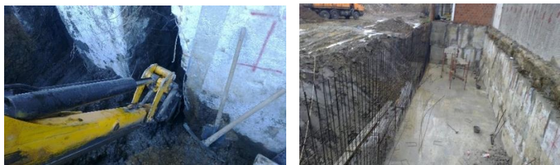
Figure 2. Under concreting and excavation of facade wall in axis 4.
