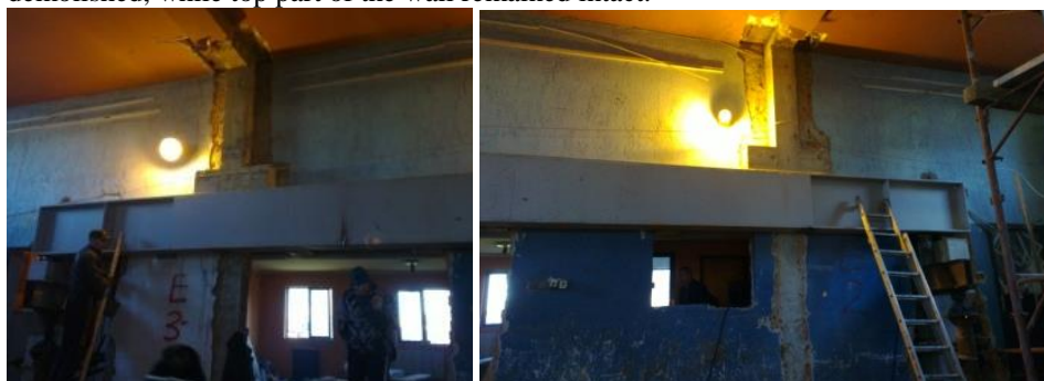
Figure 14. New short columns on top of the new steel I-beam
